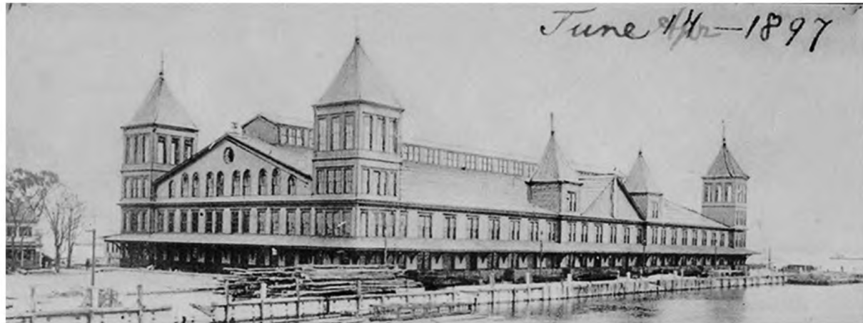
The original Ellis Island buildings were made of wood, above. After a fire in 1897, the federal government rebuilt in brick, and those buildings still stand today.
